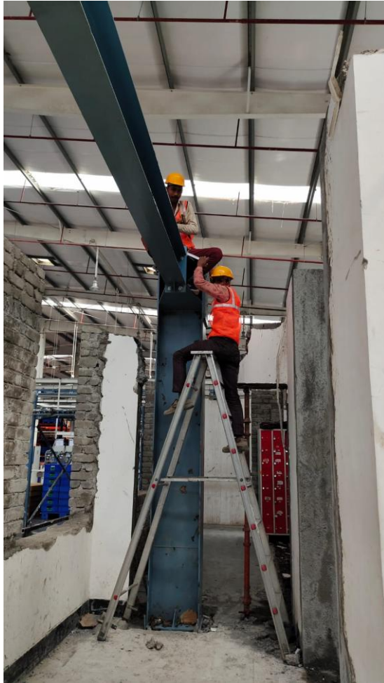
Column Erection
