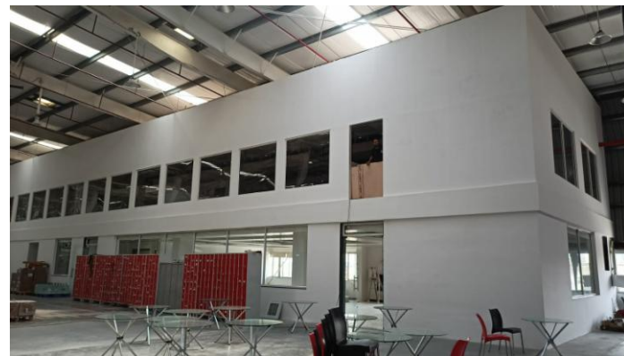
LGFS structure after completion
