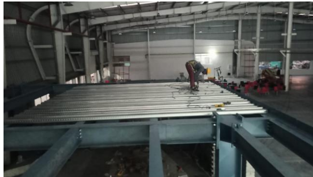
Deck slab sheet laying for mezzanine floor
