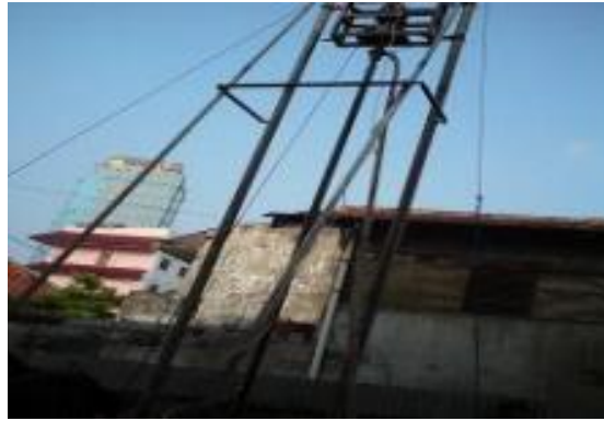
Figure 2.6 Bored Pile Gawangan
