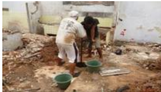
Figure 2.7 Manual Bored Pile
