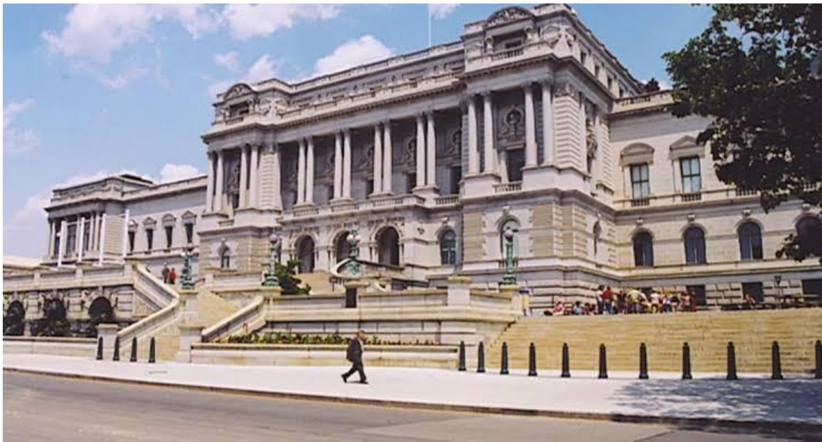
Figure 14: Front Elevation of the Library of Congress, Capitol Hill, Washington DC, USA
