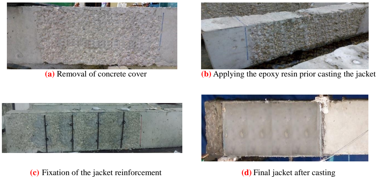
Fig. 5. Strengthening application process.
