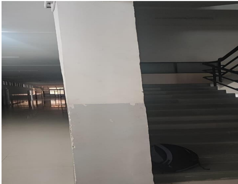
Fig.No.4.5 Undamaged Column.
