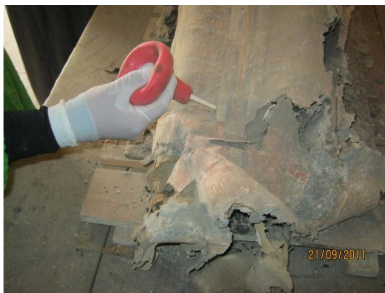
Fig.(2) describes the use of the hander air blower in the first mechanical cleaning
